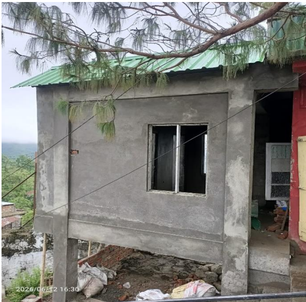
Construction of Visitor's Toilet
