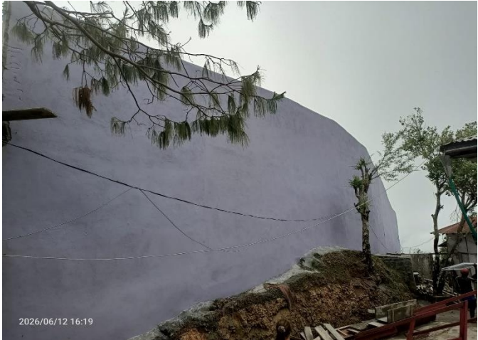
Construction of Separation Wall
