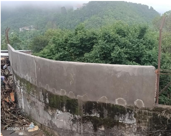
Construction of Security Main Wall
