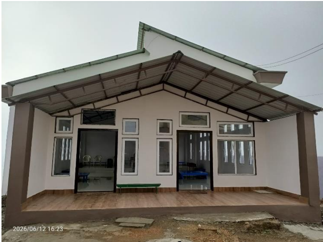
Construction of Recreation
