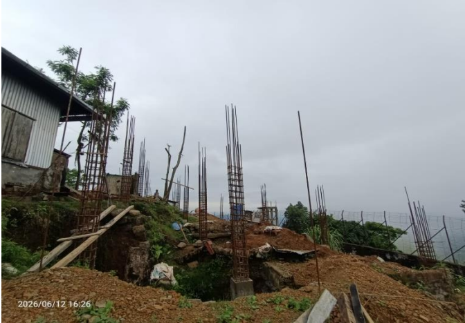
Construction of Male Ward
